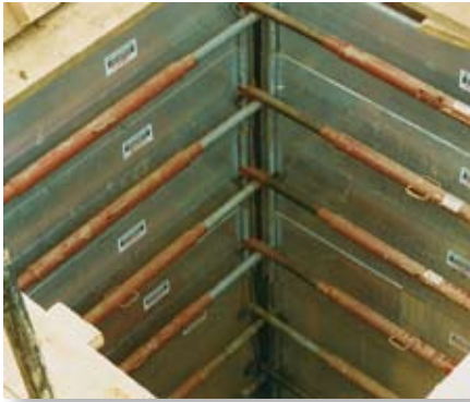
Special solution: manhole lining with additional struts
