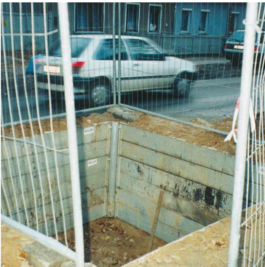
Renewal of road gullies
