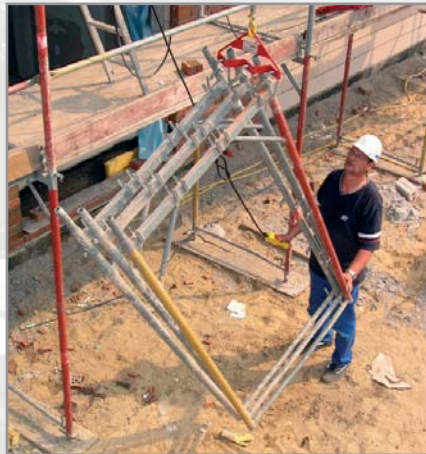
Lifting of scaffold elements
